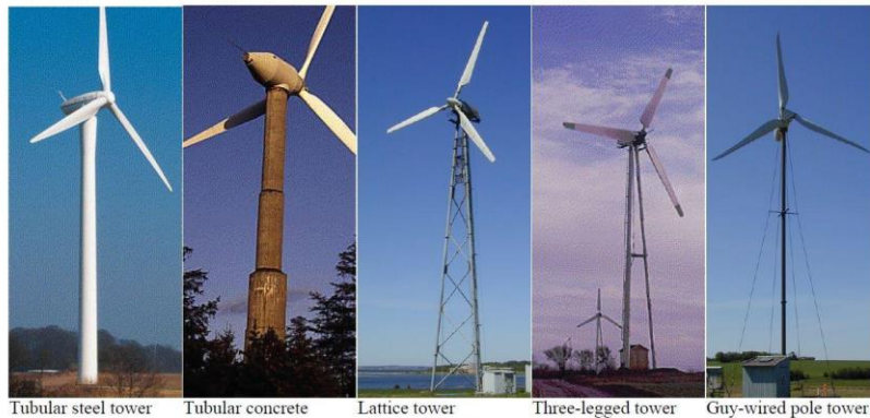
Figure 7 Wind turbines tower types [8]
