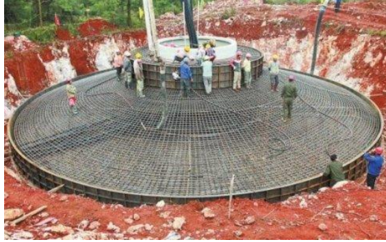
Figure 8 Onshore wind turbine foundation [9]
