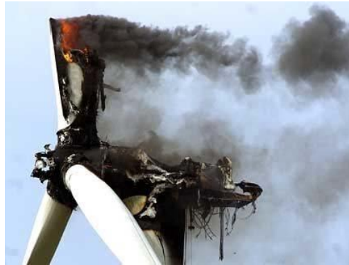
Figure 12 Geared Turbine Failure [14]
